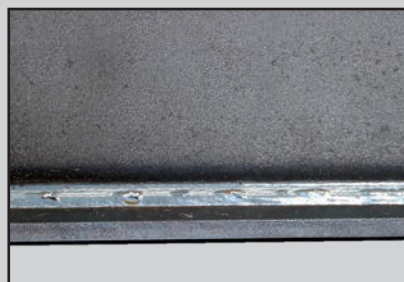
Steel fillet weld PB | 5.0 mm POWER.PULS
