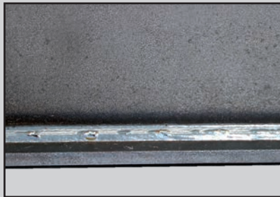
Steel fillet weld PB | 5.0 mm POWER.PULS
